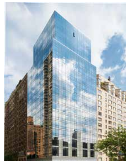
Façade din elemente Schüco cu aspect structural Schüco unitised façade as structural glazing solution
