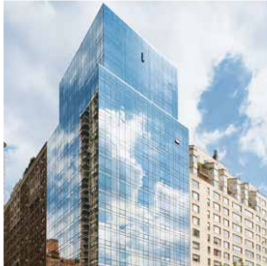
Façade din elemente Schüco cu aspect structural Schüco unitised façade as structural glazing solution
