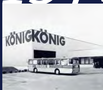
T wo warehouses as well as prototype and storage workshops for aluminum and steel constructions and steel hollow profiles are constructed in Wiener Neudorf in the industrial region of Southern Lower Austria.
